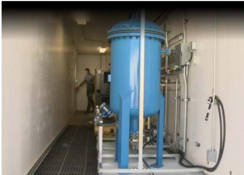
**RSL Membrane™ Housing for 10 m<sup>3</sup>/hr in a 6 m trailer**
